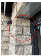
Mortar cracked
