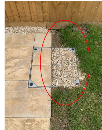
Poor appearance gravel could get in mower
