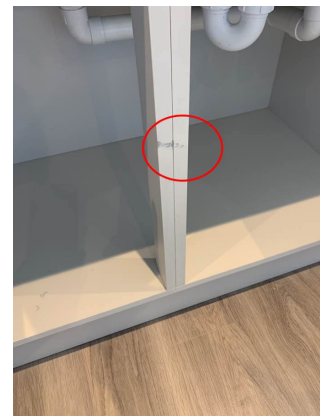
Clean off paint
