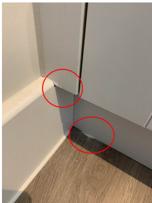
Clean off paint
