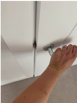
Latch doesn't retreat against the strike plate
