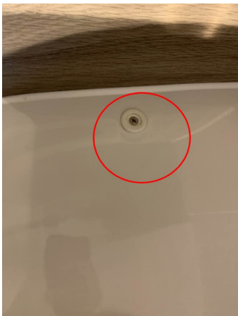
Cap missing side of toilet
