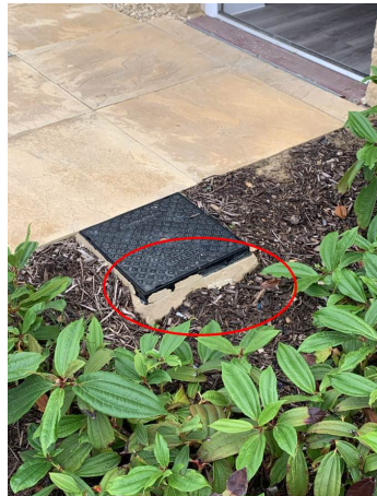
Cement pour around chamber cover
