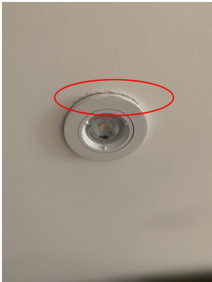
Make good around down lights
