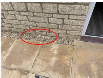
Air brick below ground level
