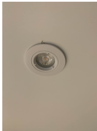
Make good around down lights
