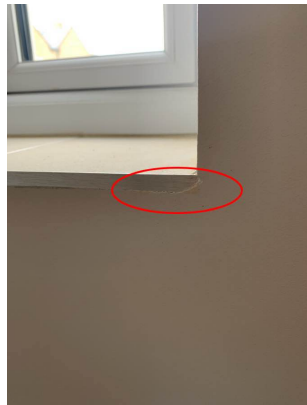
Make good around sill tile trim
