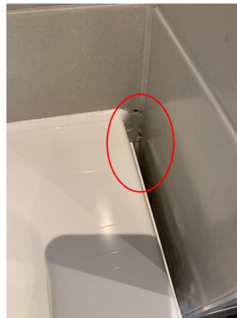
Poor finish by right end of bath
