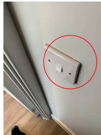
Make good around switches/sockets
