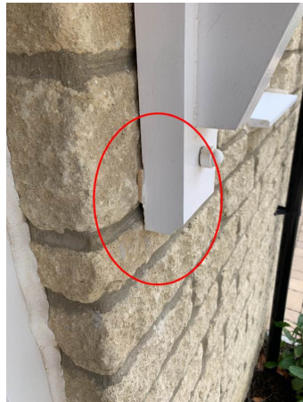
Spacer protrudes behind bracket
