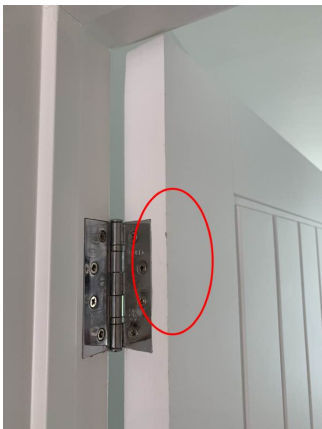
Touch up doors throughout house
