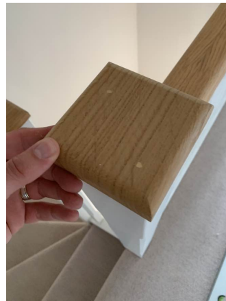
Make good fixing holes on caps
