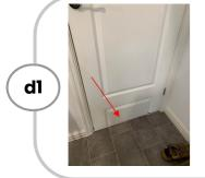
Unsightly cut door - excessive cut can have adverse effects on door structure
