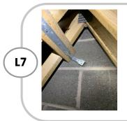
The restraint strap should be connected to the inner leaf of the blockwork  ${\mathbin{\triangle}}$  Significant issue
