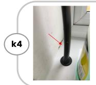
The sealant around the window is poor and need redoing
