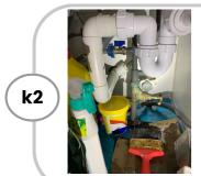
In April 2017, the Water Regs UK changed the installation requirements of the Water Supply (Water Fittings) Regulations 1999. At the point where an appliance, such as a dishwasher or washing machine, is connected to the water supply, it will need an additional DCV installed 🛆 Significant Issue
