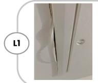
There is a gap around the loft hatch to caulk for a neat appearance
