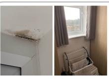
Mould at window reveal - likely condensation
