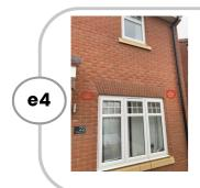
The weep vents have inconsistent spacing: they should be in 450mm apart according to NHBC 6.1.17  ${\rm \triangle}$  Significant issue
