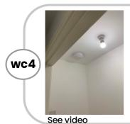
The extractor fan should overrun by 15 minutes due to there being no window, as per Building Regulations part F 🛆 Significant Issue
