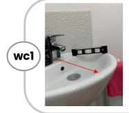
The sink is not level which may be an installation or manufacturing defect
