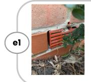
The air brick is damaged and needs replacing
