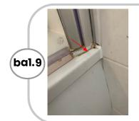
There is missing sealant. Mastic trade to fill with moisture resistant sealant
