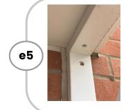
The gallows brackets are missing fixing covers to protect / improve appearance
