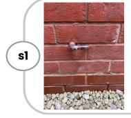
Boiler pressure relief valve pipework should be vertical
