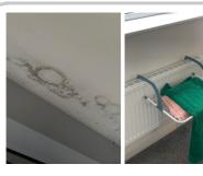
Mould at window reveal - likely condensation
